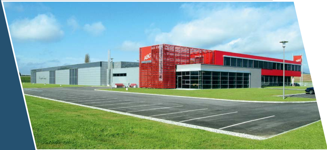
Zentrale Klagenfurt Headquarter Klagenfurt
